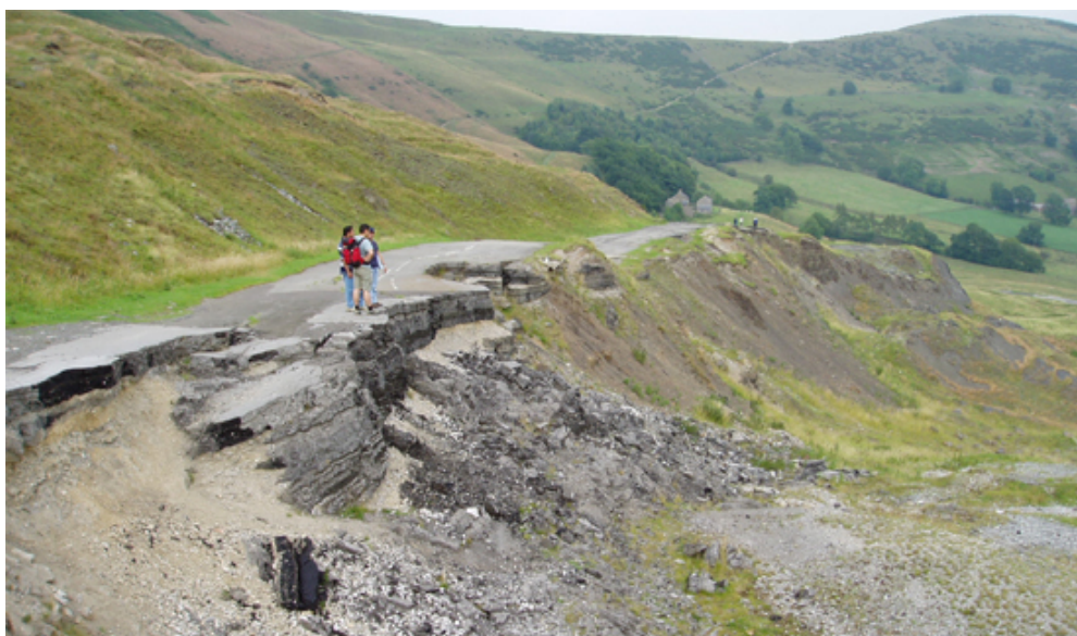
Collapsed road beneath Mam Tor (Credit: British Geological Survey)
